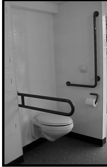
Figure 2. Lavatory with knee access Figure 3. Wall-hung toilet; grab bars Figure 4. Small transfer shower
